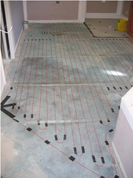
Run the cable around to the opposite side of the heated space, then zig zag the cable back towards the termination point sticking down at the ends only until you are satisfied that reasonably even spacing is achieved. Then apply further strips of tape across the runs at about 400mm spacing.
