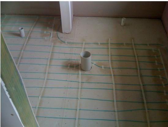
Unroll the cable rather than pulling it sideways in loops, as this will form twists. Take care not to apply unnecessary tension at any time, especially at the end joins. When nearing the end, you may find it necessary to make minor adjustment to spacings in order to finish up where you intended.
